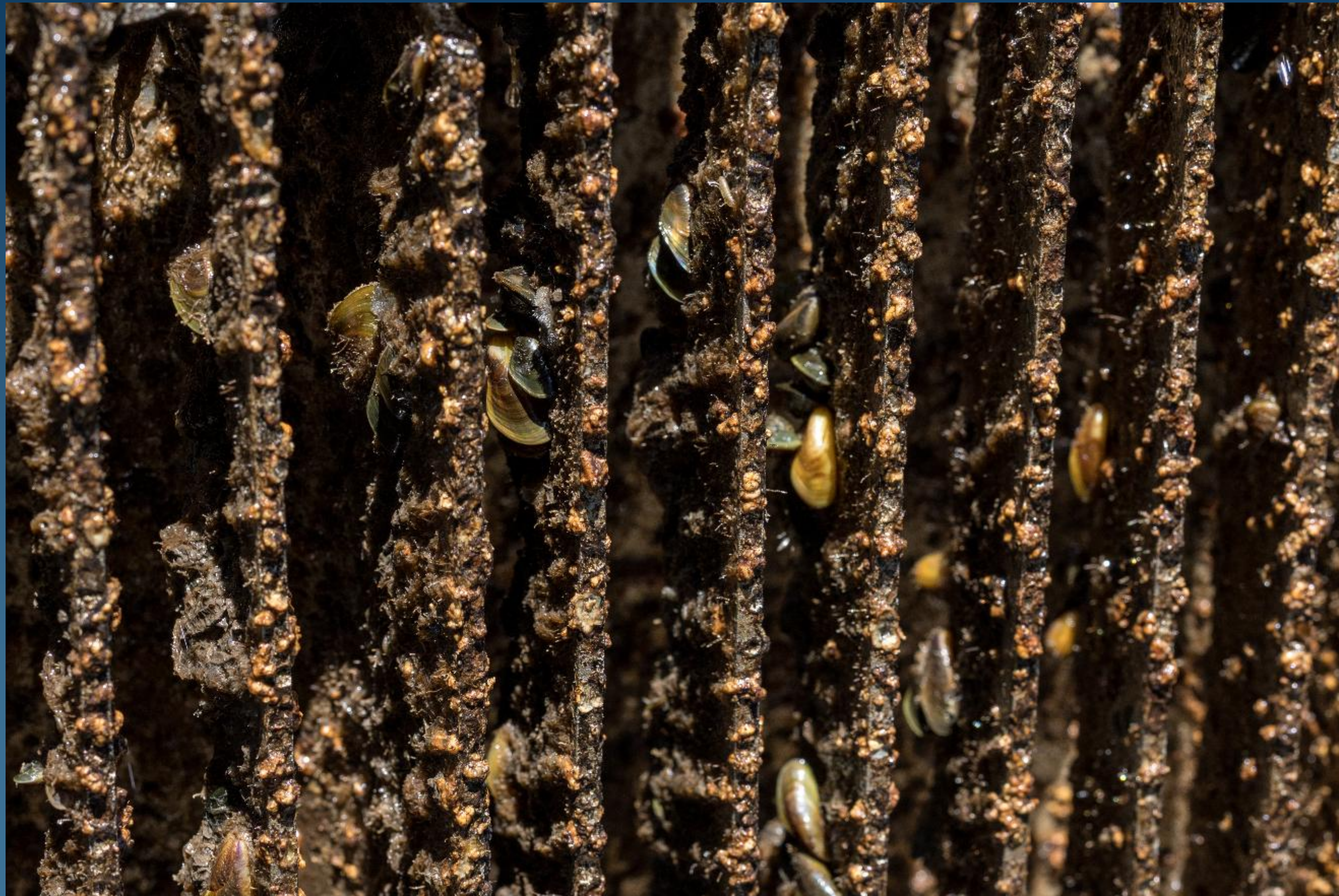
Golden mussels attached to Skinner FF louvers 07.01.25
