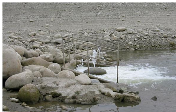
Figure 2.21: Turnout Facility at Azusa
