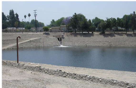
Figure 2.20: Turnout Facility at Irwindale
