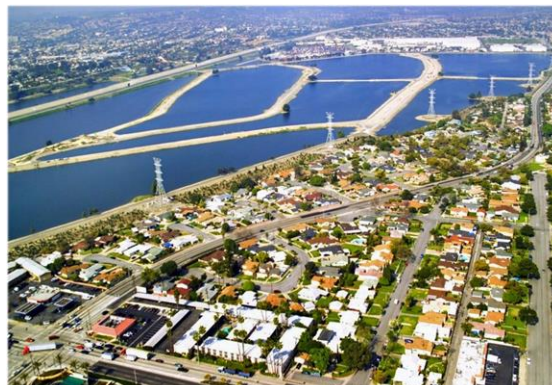
Figure 2.9: Rio Hondo Spreading Grounds
