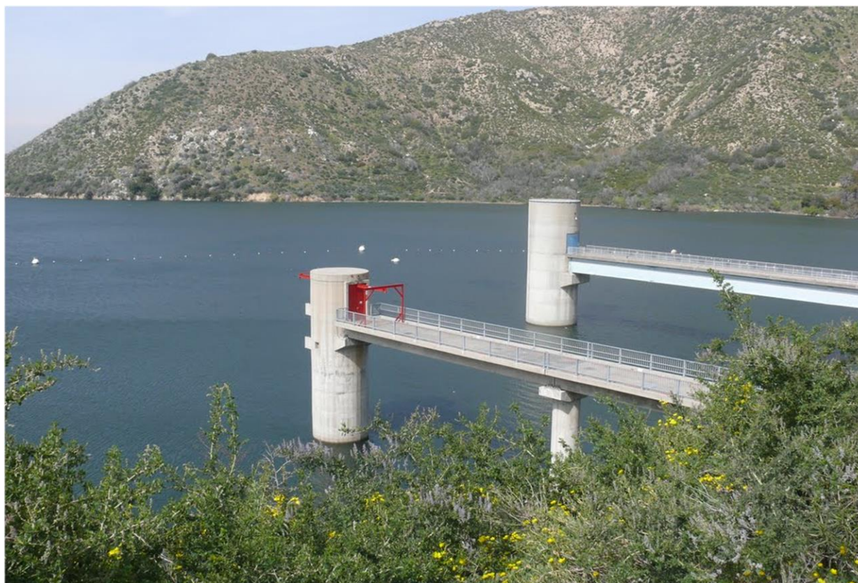
Figure 2.4: Intake for Devil Canyon Plant at Silverwood Lake (part of SWP's East Branch)
